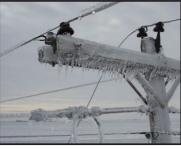
large transformer. Strong high winds and ice that accumulates on lines can also impact distribution.
